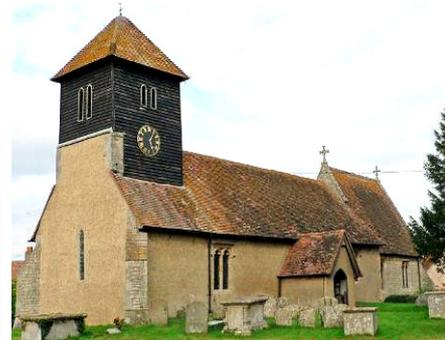
The tower is unusual being a largely independent timber structure within the west end of the church. All towers move when bells are rung – however the movement here was not ideal because
